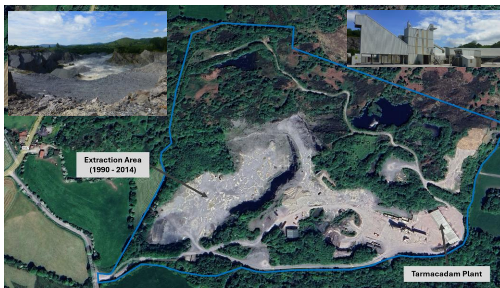
Figure 1: Aerial image of Ardcahan Quarry and macadam plant within the applicants landholding (outlined in blue). Extraction area and macadam plant also shown inset
